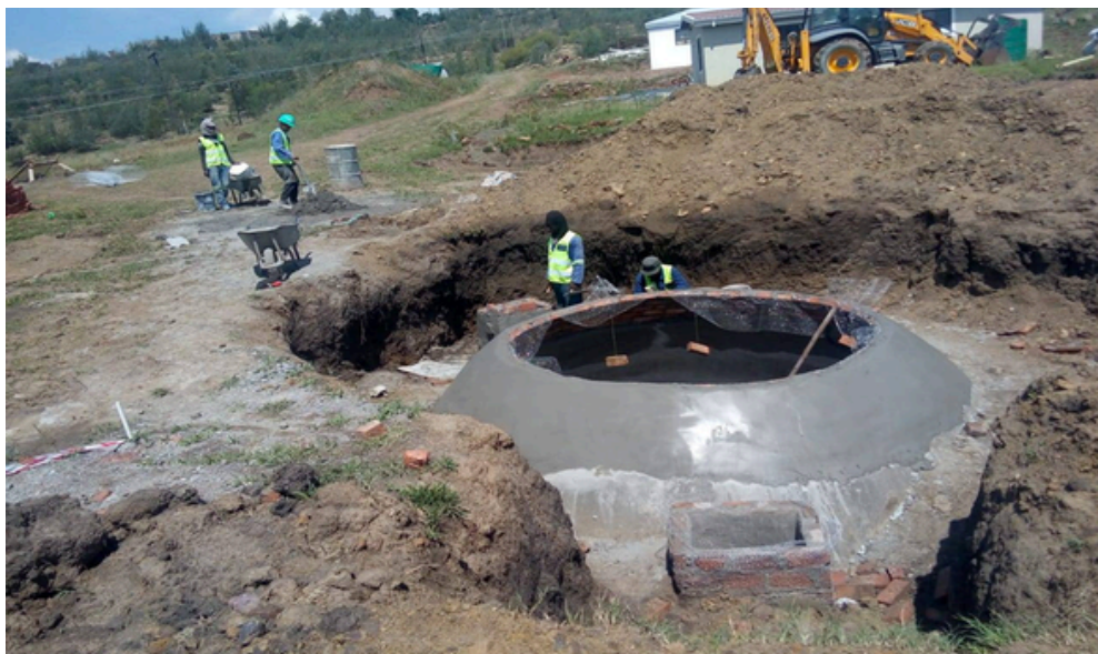
Figure 9: Biogas digester under construction by Kaeane Renewable Energy Developers.
