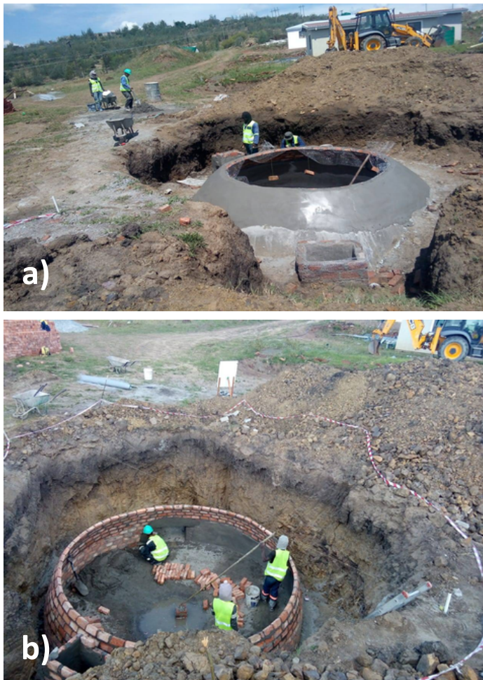
Figure A5.2 a & b: Biogas digester under construction by Kaeane Renewable Energy Developers.
