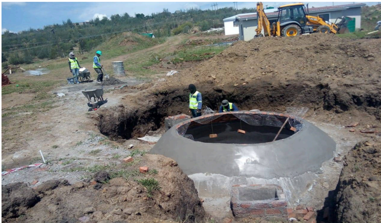
Figure 4: Biogas digester under construction by Kaeane Renewable Energy Developers.
